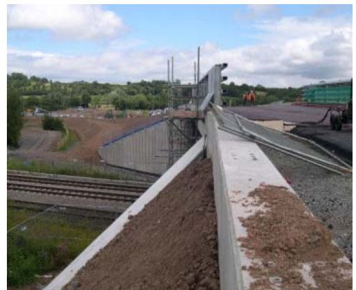
New Leominster railway bridge nearing completion.
